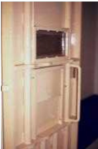
Figure 5 Metal inner cell door with window and speaking grille
